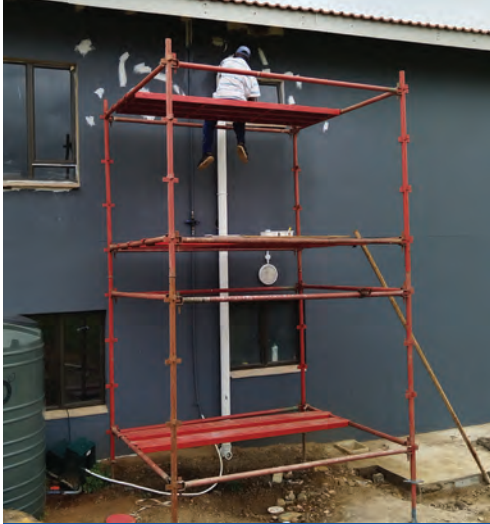
Wiseman painting and being supported by Form Scaff's scaffolding
